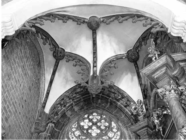
Figure 9. Wrocław Cathedral, vault of the Holy Trinity Chapel, 1390s (photo: author).
