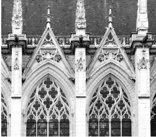
Figure 19. Vincennes, Sainte-Chapelle , window tracery in the nave, ca. 1400–1410 (photo: author).
