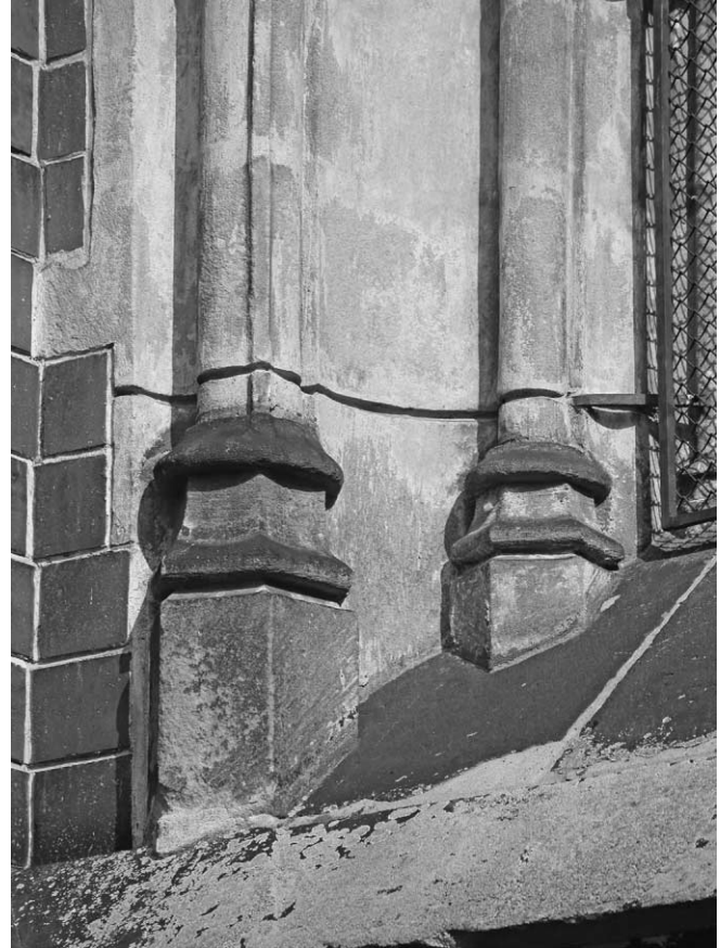
Figure 12. Legnica, parish church of Saints Peter and Paul, plinths of external tracery mullions of the von der Heyde Chapel, 1420s (photo: author).
